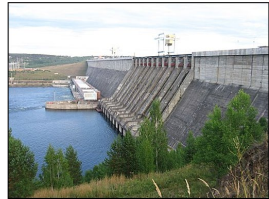
Ust'-Ilimsk HPP Reservoir 1922 km 2
